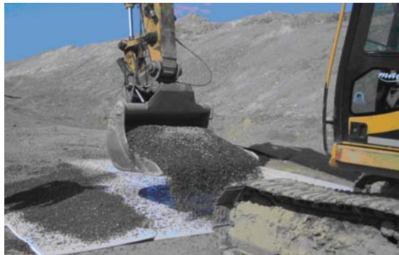
Figure 4 – Installing XPS insulation boards
