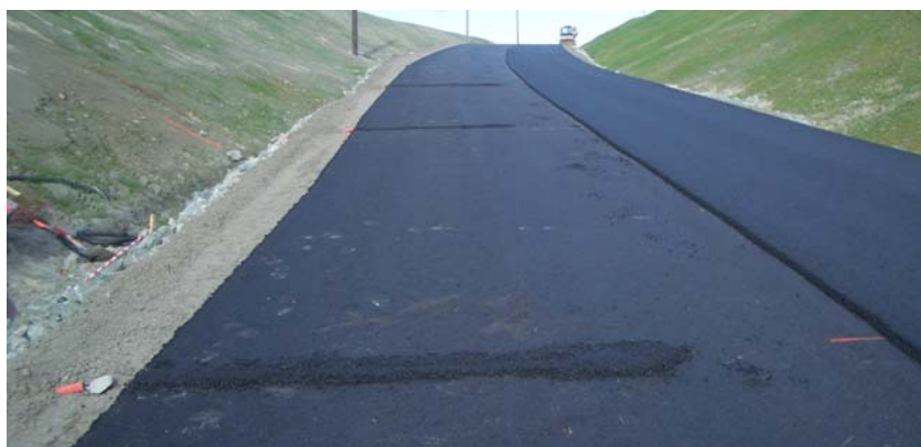
Figure 7 –temperature sensors between asphalt layers
