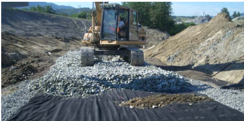
Figure 6 – Separating geotextile, covering with crushed rock
